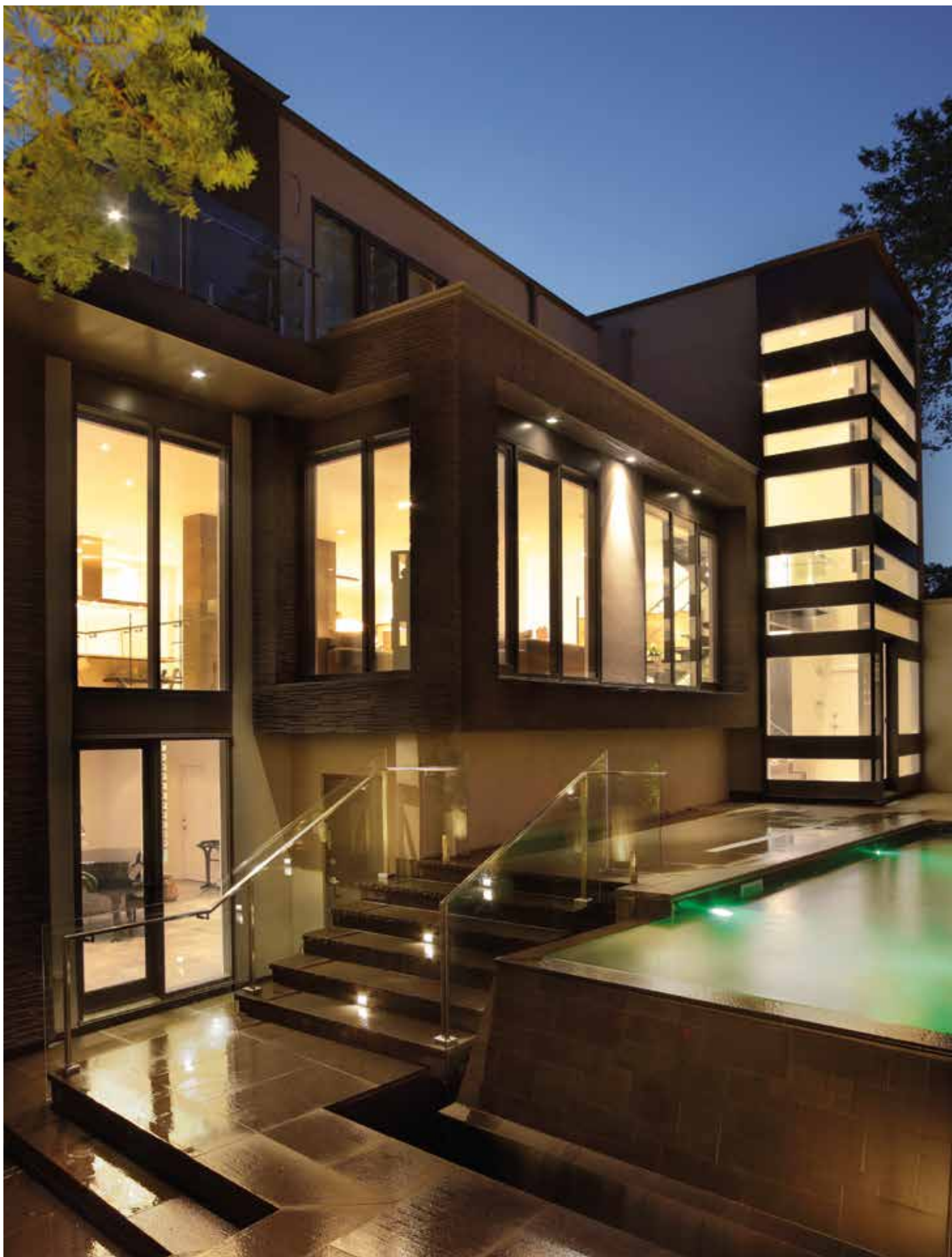
EXTERIOR LIGHTING WALL LIGHT - Recessed
