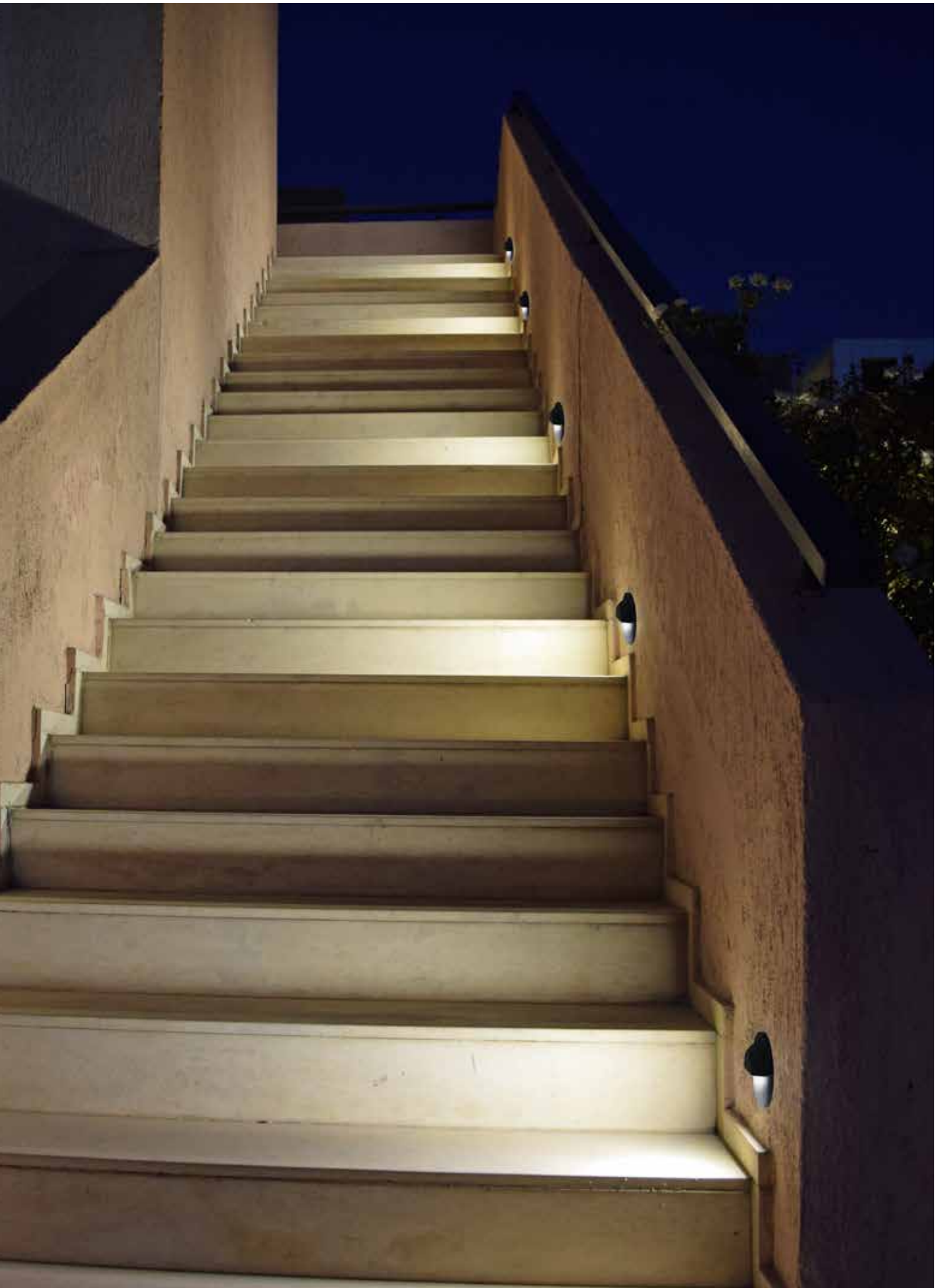
EXTERIOR LIGHTING WALL LIGHT - Recessed
